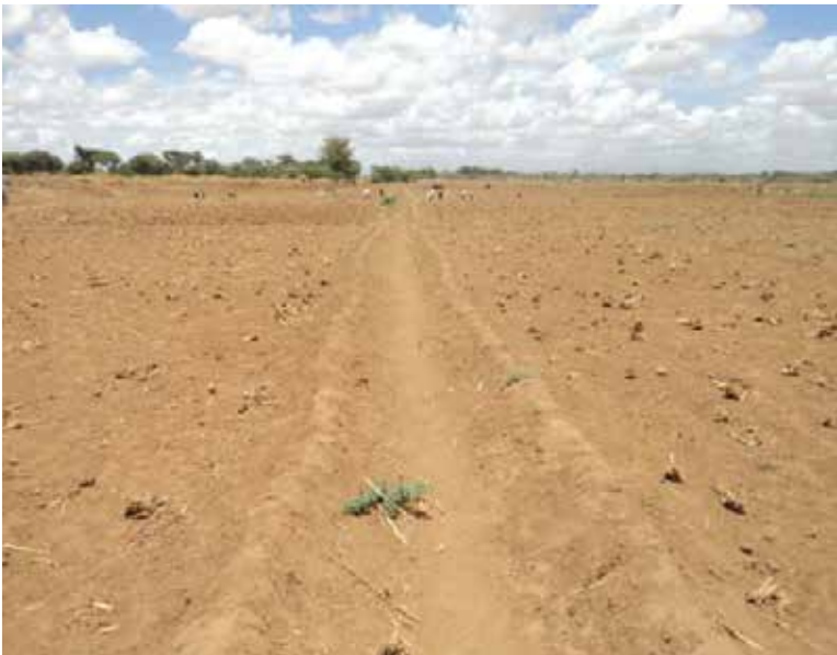
Plates 2 and 3: Vegetation clearing and land leveling to create conducive irrigation environment at Katilu and Nanyee irrigation schemes in Turkana County (Photo: Jesse Owino)
